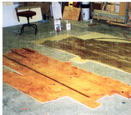
2. The two panels, ready to glue
