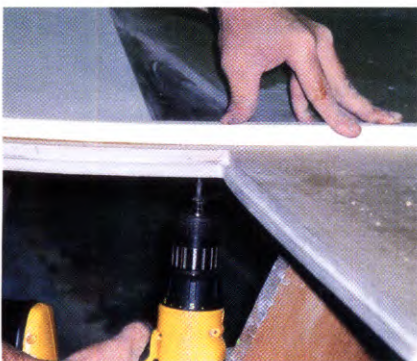
13. Removing screws from border
