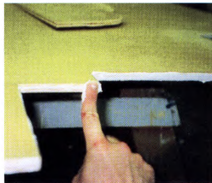
5. Sealing the edges of the panel with paintable acrylic caulk
