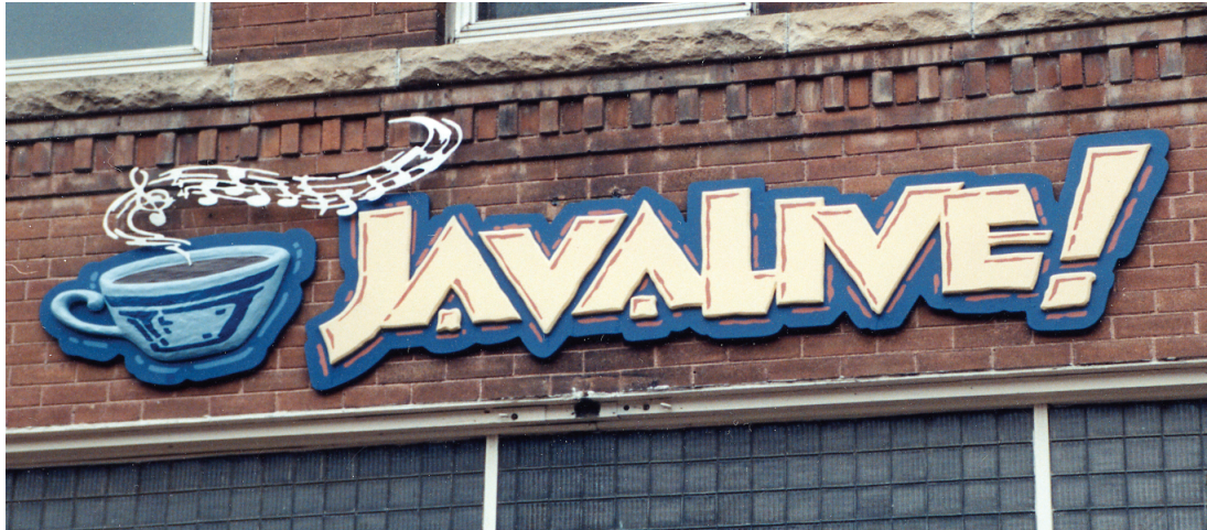
High-density urethane board lettering and coffee cup mounted on a 3-by-12-ft. panel of 1/2-in. overlaid plywood, finished with acrylic paint; cutout music notes are .080 aluminum
