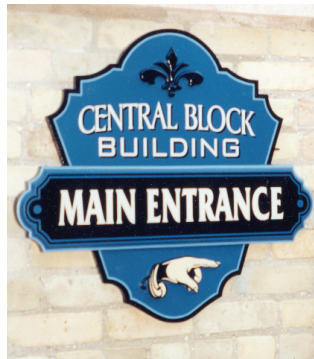
Vinyl lettering on 3/4-in overlaid plywood panel, finished with acrylic latex paint; Main Entrance panel and carved hand are high-density urethane board
