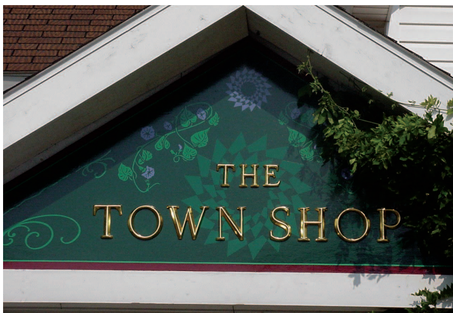
Gold-leafed Gemini letters [www.signletters.com] on aluminum composite material painted with OneShot bulletin enamel
