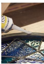
After the desiccant was added to absorb any ambient moisture, the unit was sealed air and water tight with silicone and then screwed shut. To date, we've had no fogging!
