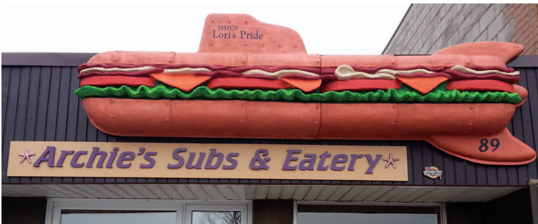
The sub is 4-by-13-ft. coated foam on overlaid plywood and the sign is a 2-by-10-ft. Extira panel.
